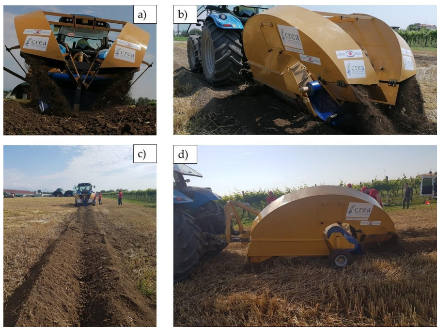
Figure 3 Rear view of the prototype. b) Prototype while working. c) Vision of the soil after the installation of the SWRS. d) Lateral view of the prototype.
